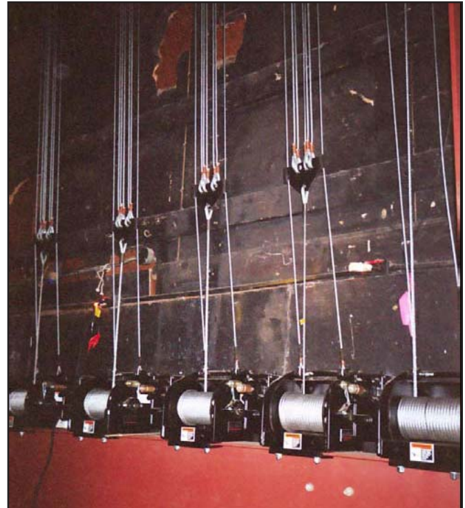
A row of Thern clew winches hold set lines in place at the Diamond Head Theatre.
