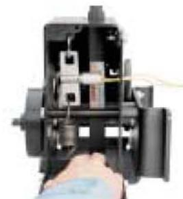
The test arm is pulled down to release the fire vent doors without breaking the ETL<sup>®\*</sup>.
